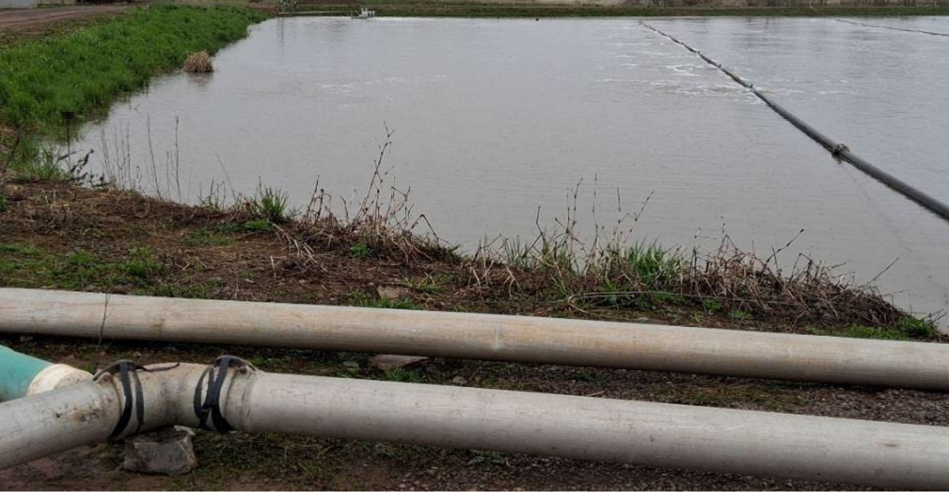
Temporary yard piping installed to transfer water from healthy lagoons to Lagoon 1
